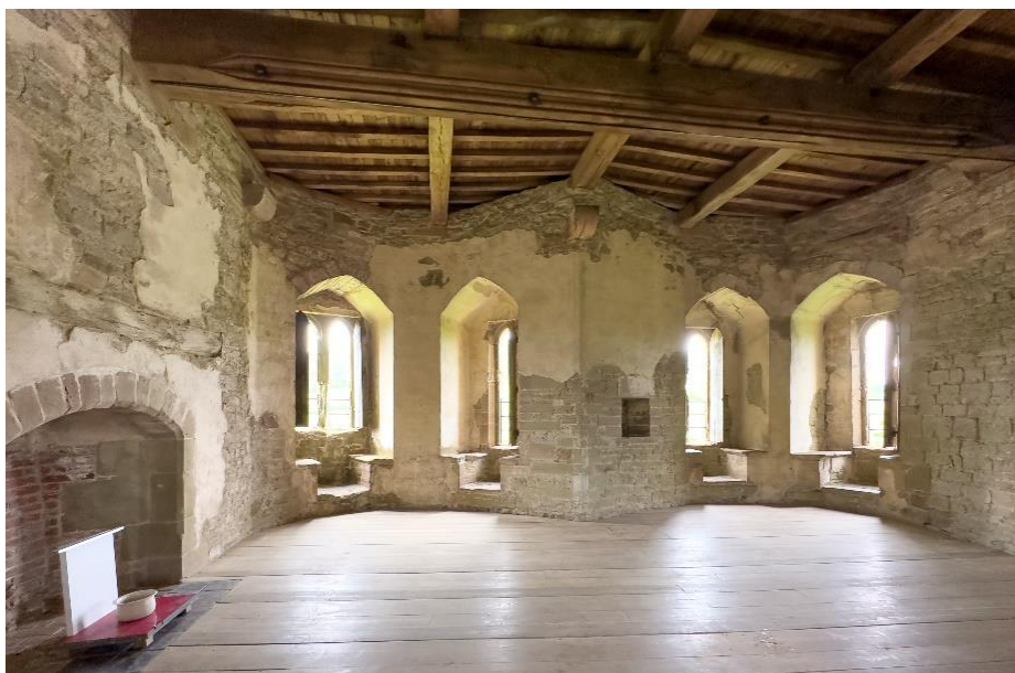
Inside the south tower (photo by Alan Santillo)
