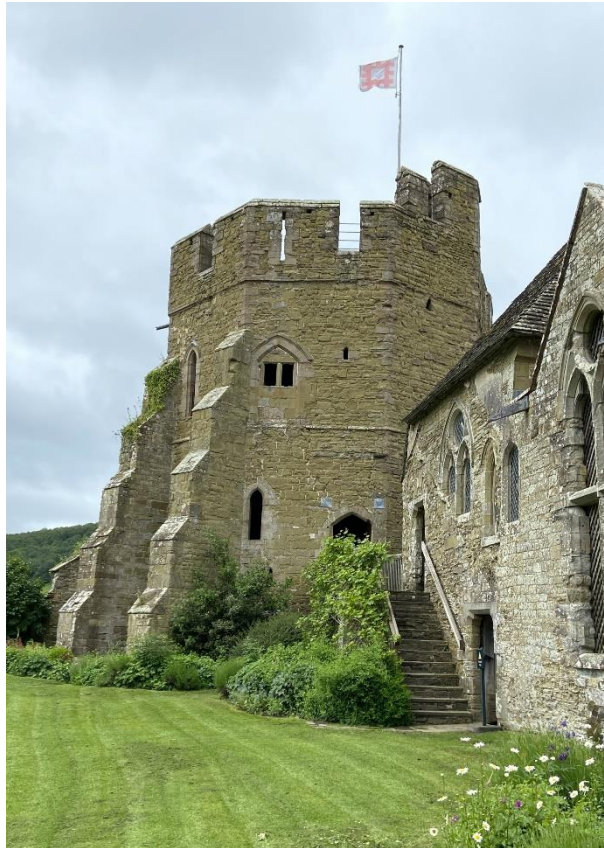
The handsome south tower exterior
