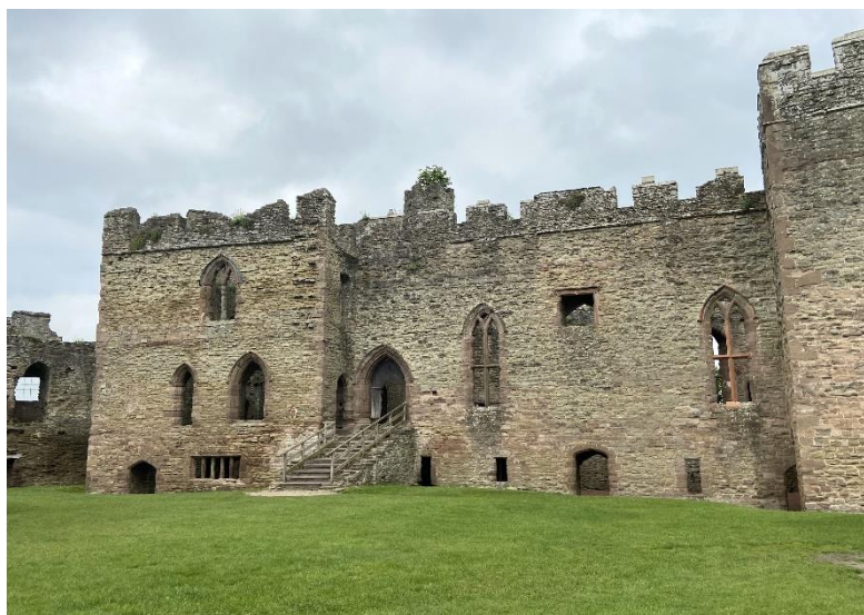
The solar block
