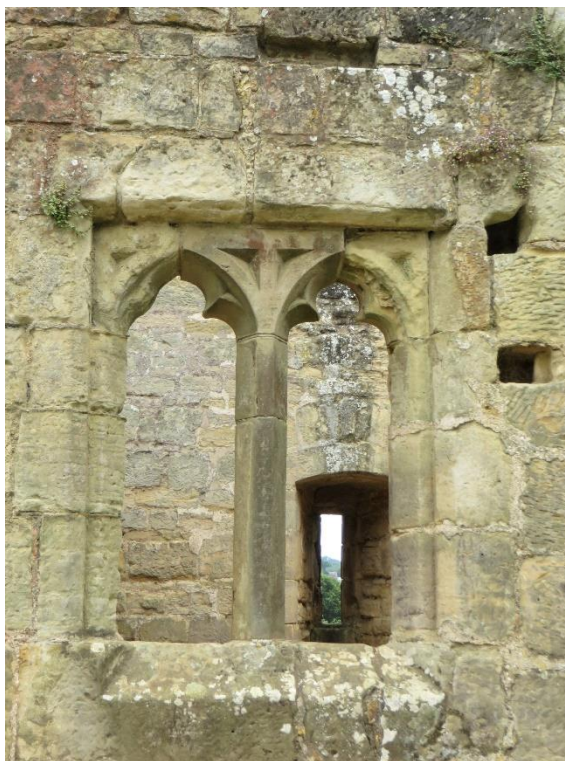
Withstanding the test of time
