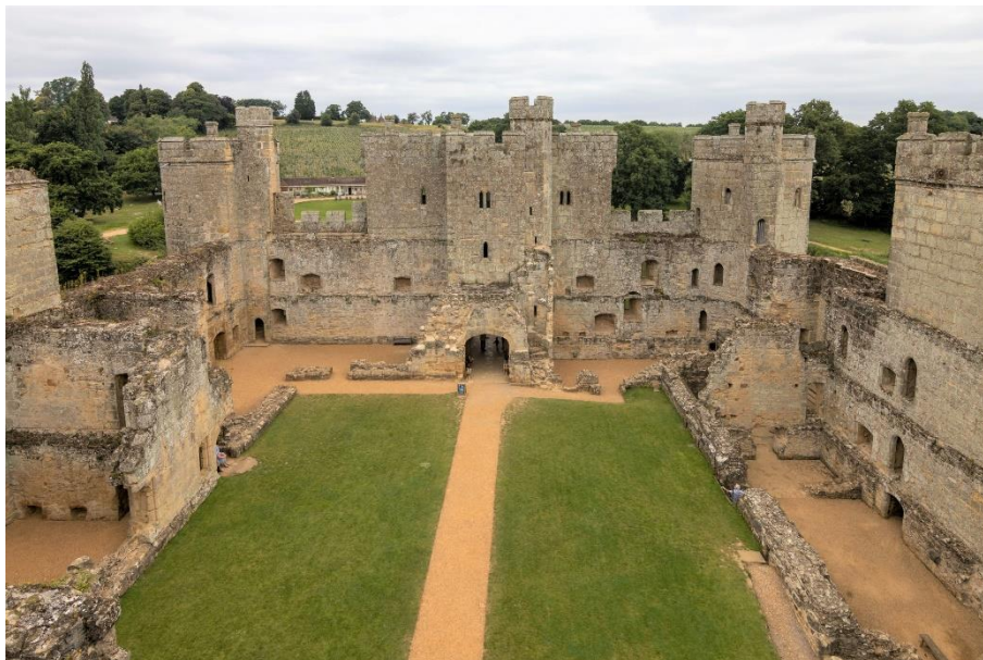
View from the postern tower (photo by Alan Santillo)
